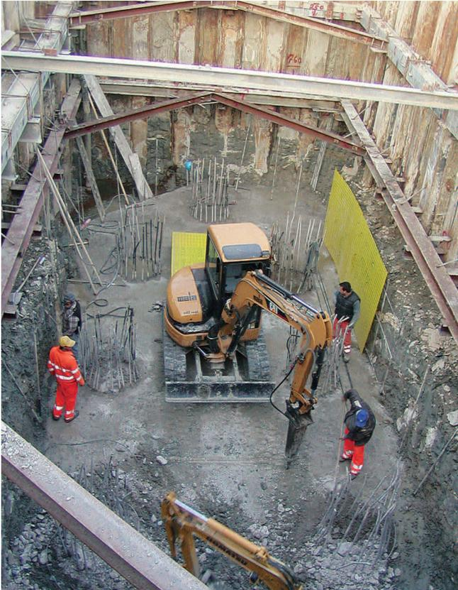
Photo 6 - The excavation pit of the pier 9 foundation.
