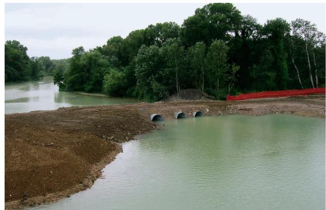
**Photo 5 - The cofferdam of the pier no. 9**
