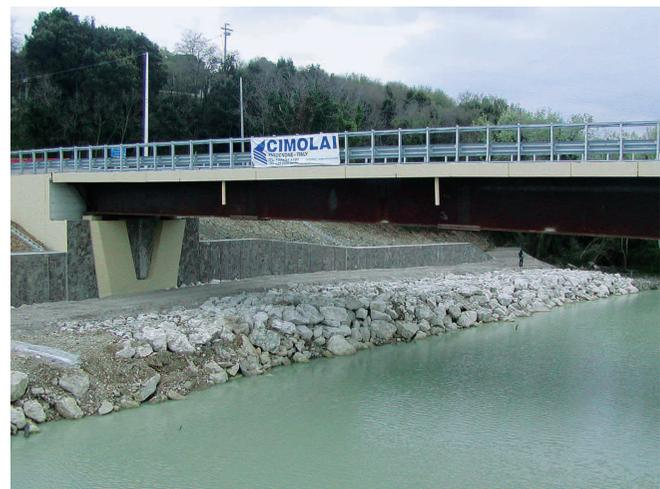
Photo 7 - Riprap revetment on right river bank.
